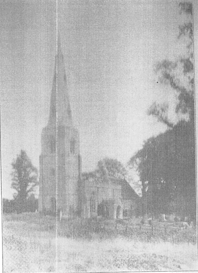
BRINGTON CHURCH FROM THE SOUTH-WEST
