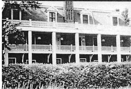
In the 1940s, the structure of the porch was altered.
