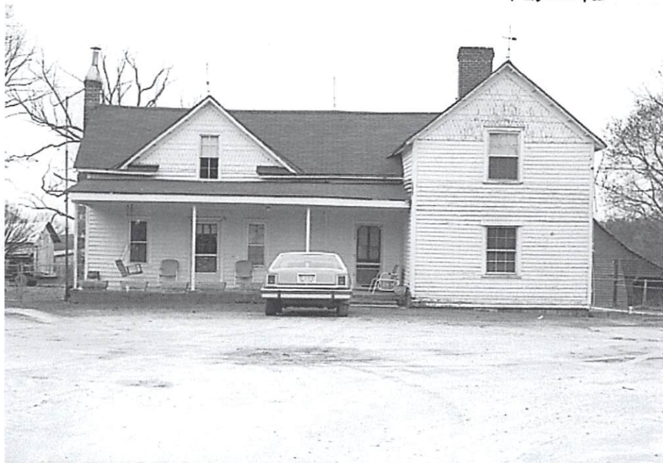
GREEN LVL CH RD, W/NC JOE JOHN YATES HOME (35) DESTROYED
