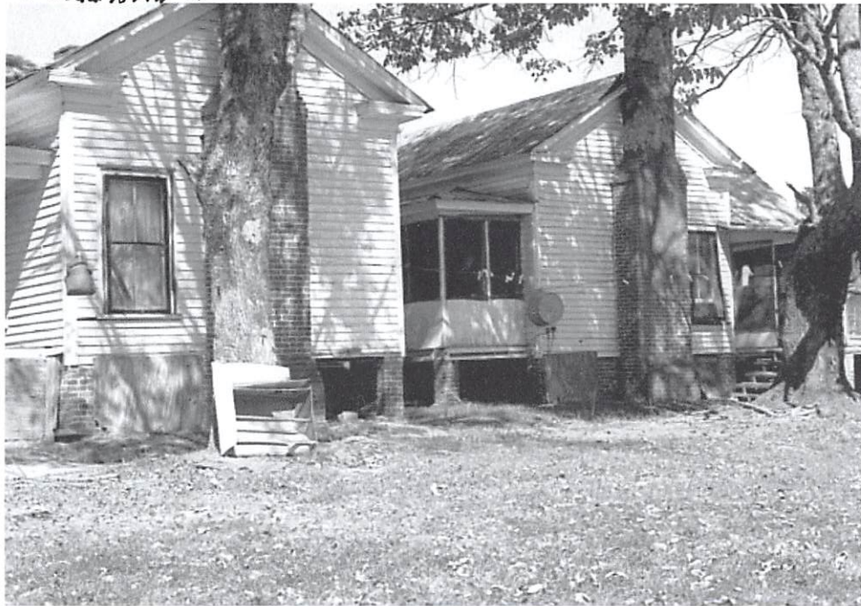
OLD PLACE RD, WAKE CO, NC DESTROYED (27) HILLIARD & KIDDY BATHGELOR YATES HOME
