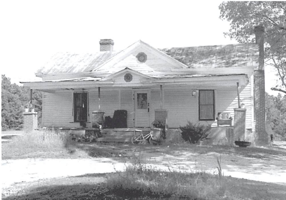
OLD PLACE RD W.C., NC HILLIARD & KIDDY BATHGELOR YATES HOME DESTROYED (26)
