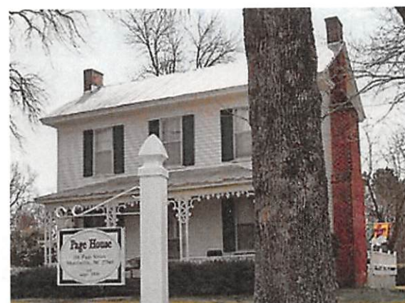
(July 2007) The Page house survived the fighting at Morrisville, however the marks from bullets and shells are visible on the chimney nearest the railroad tracks
