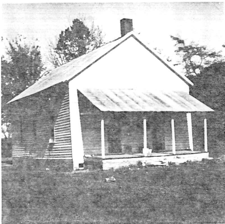
A one-room school building, typical of many once found in Bollinger County.
