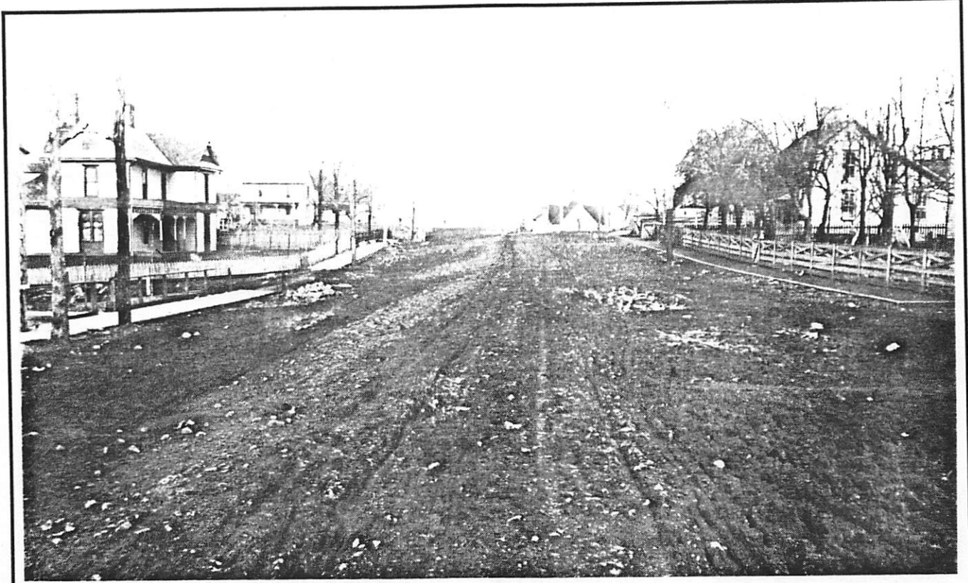
VIEW OF PIKE LEAVING TOWN SOUTH - MARCH 28, 1907
